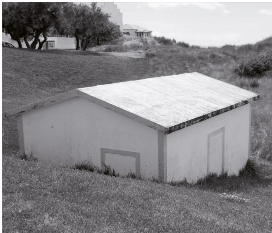
▲ Cable House, where the submarine cables were tied, in Porto Pim Bay, Faial, Azores (June 2017). Photo by: Joana Gaspar de Freitas.
